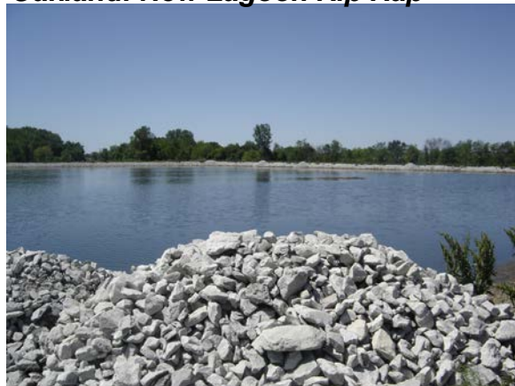
Oakland: New Lagoon Rip Rap
