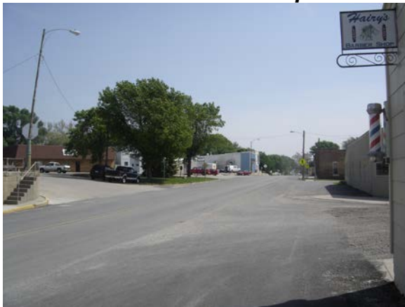
Minden: Tamarack Road Improvement
